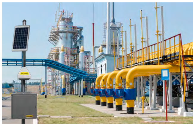
Figure 1. The GAZPOD monitoring station measures on a continuous basis up to four gases simultaneously. Monitoring data is transferred via wireless cellular connection to an enterprise management system for storage and processing.
